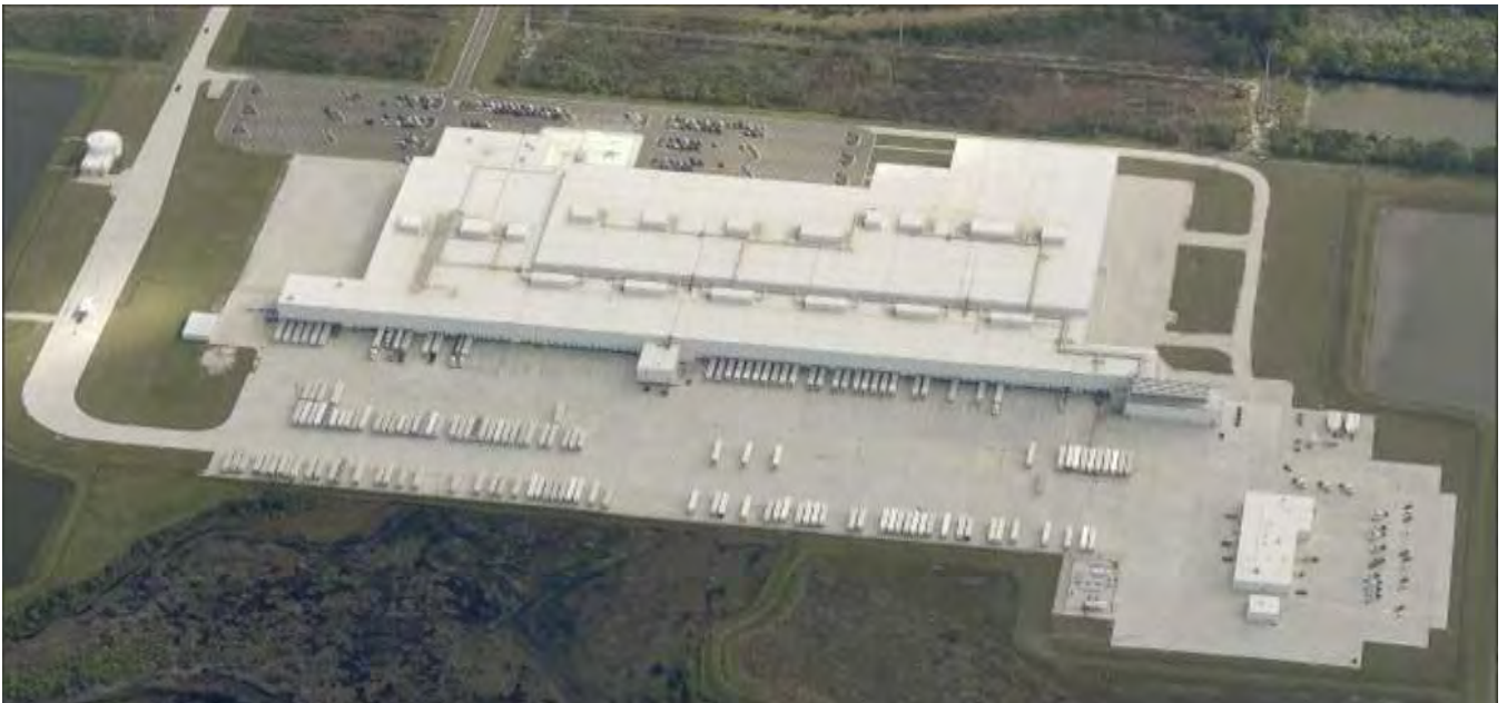
Figure 10-13.5 Walmart Cold Storage and Warehouse Distribution Center
