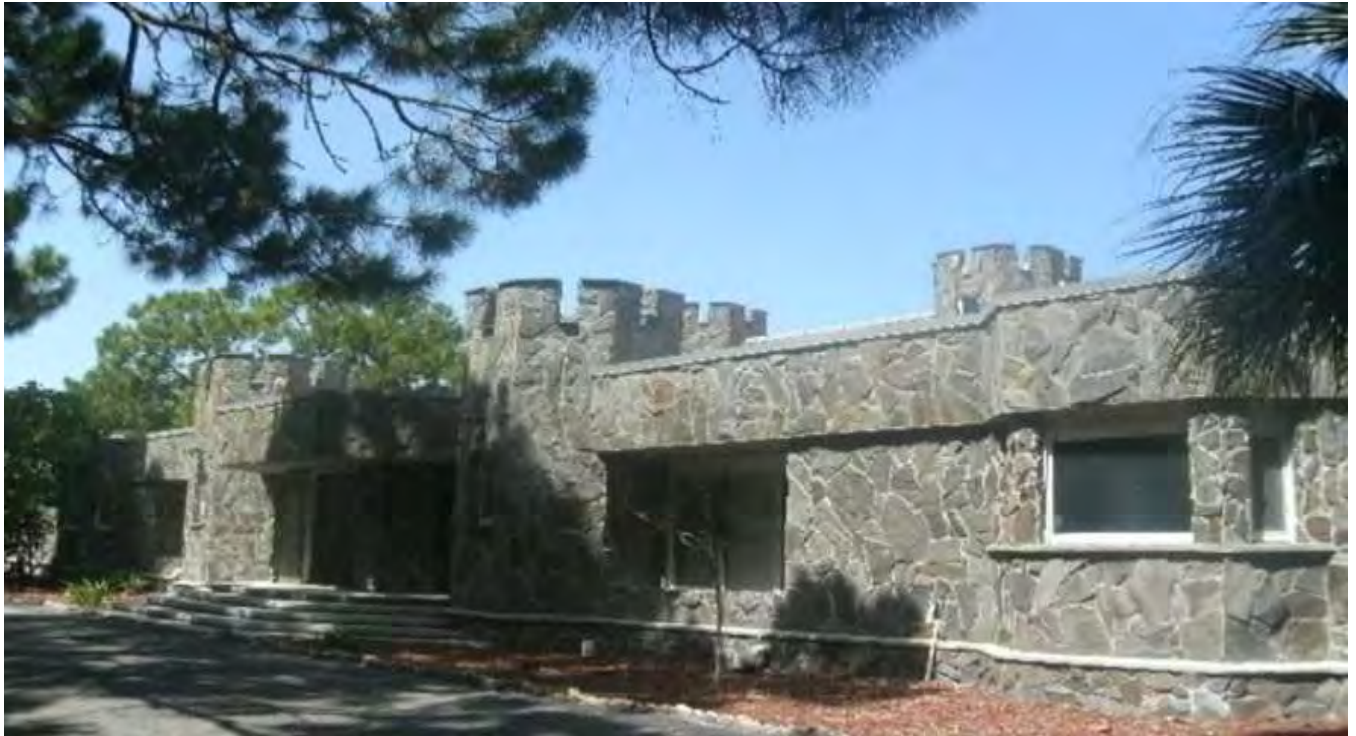
Figure 9-6.1 “Castle” Home with Functional Obsolescence
