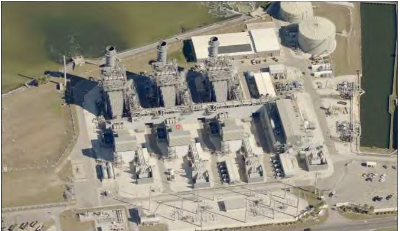
Figure 11-3.1 Florida Power & Light's Natural Gas Cape Canaveral Clean Energy Center
