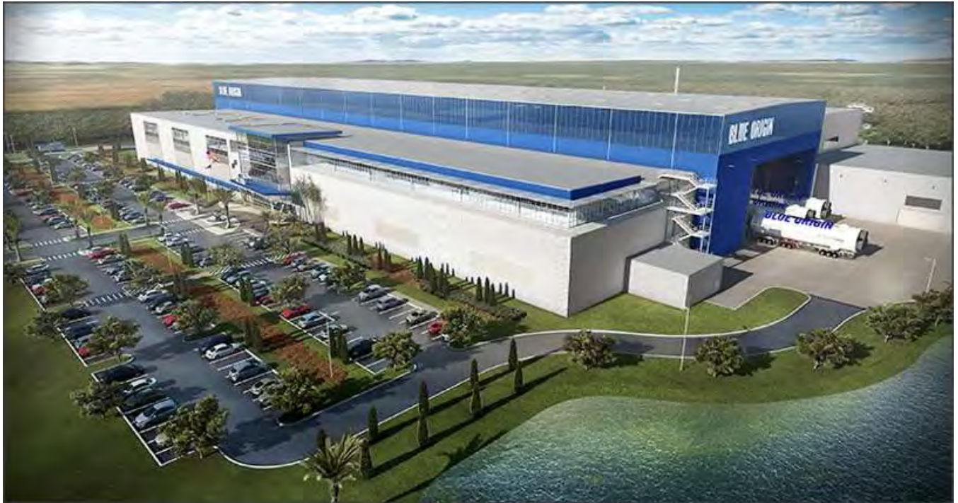
Figure 10-13.2 Blue Origin Aerospace Facility
